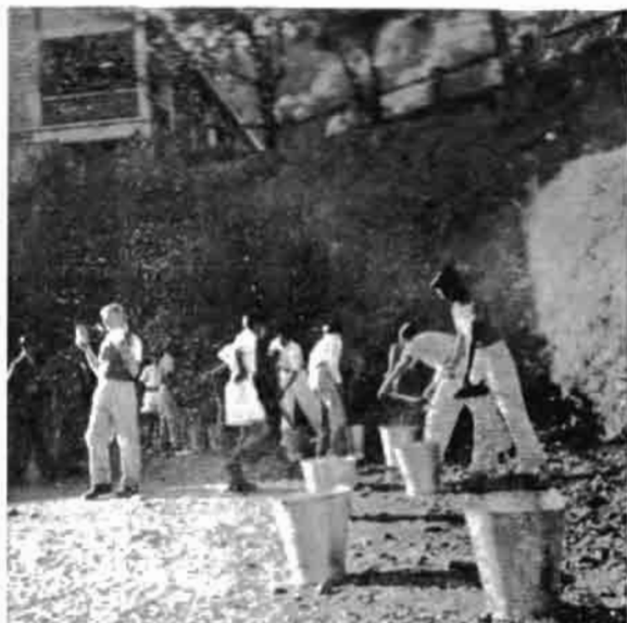
Working on the Swimming Pool.
